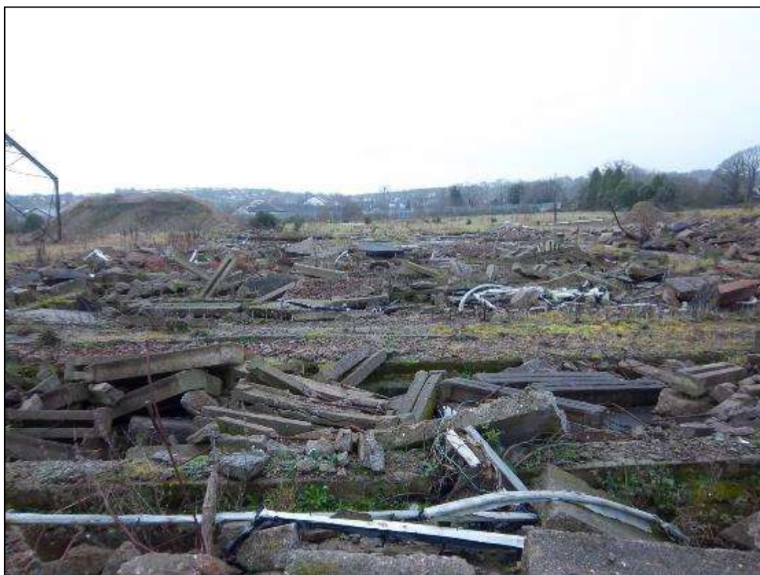
Plate 13.18: Central area of brownfield site; looking south-west.
